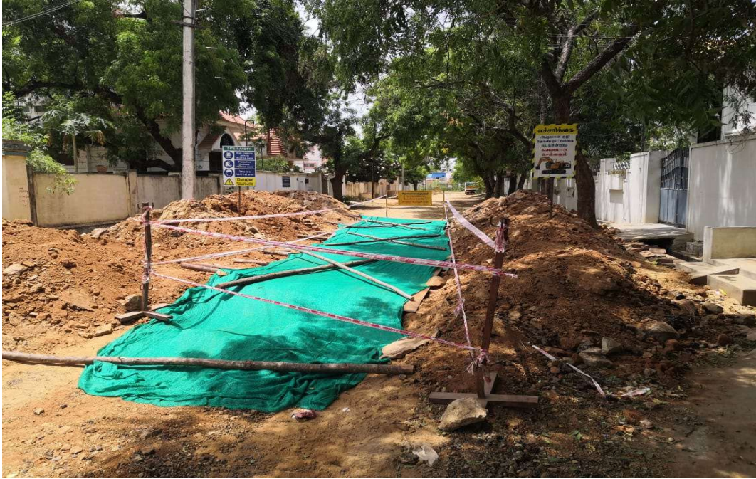
Proper coverage of trenches with MS sheets and shade net
