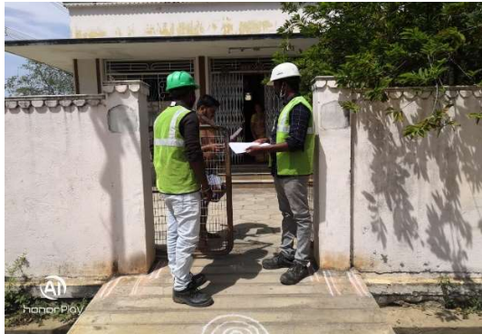
Issue of Prior Notice to the Public in the nearby Blasting area
